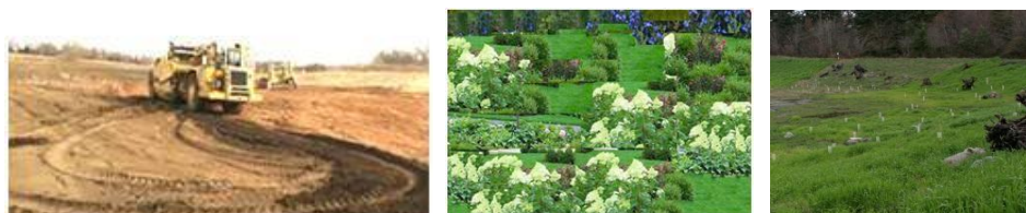
Figure 4. Borrow pits filled and rehabilitated
